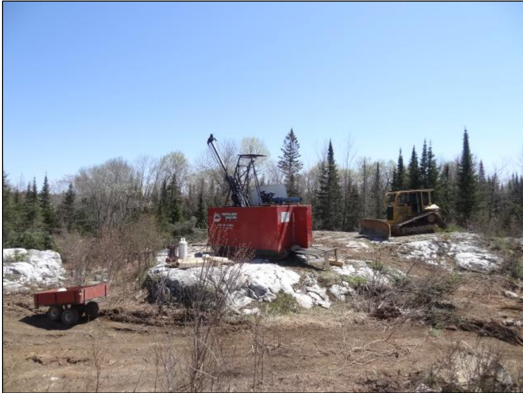
Figure 10.3 Drill Set-up During the M.Plan May, 2018 Site Visit
