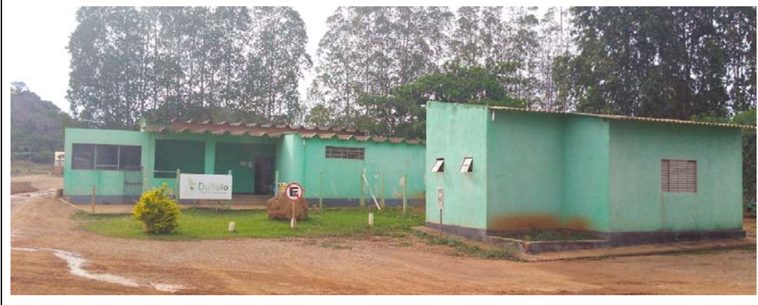
Figure 18.3_2 Office Installations at the Processing Plant
