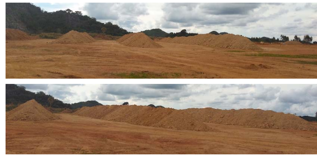
Figure 18.3_3 Run Of Mine Material Stored on the Lot of the Processing Plant
