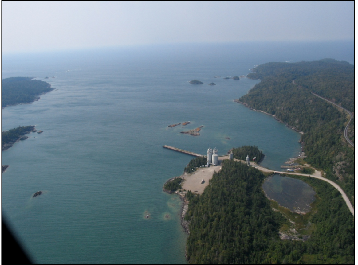
Figure 5-1: Heron Bay Deep Water Harbour and Infrastructure
