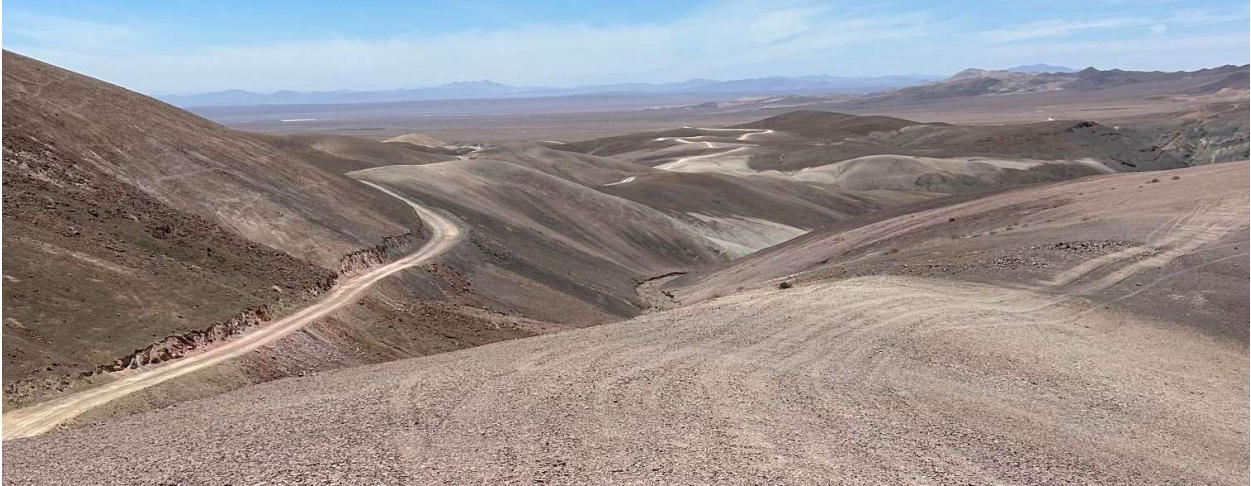
Figure 2: Portion of newly constructed 5.2 km access road into Cerro Blanco
