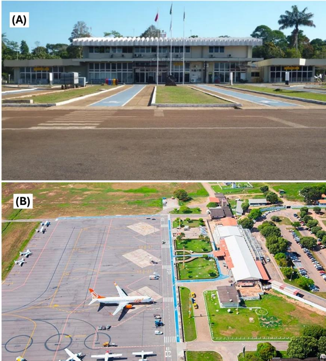
Figure 5-3: A) Carajás Airport building view. B) Marabá airport aerial view
